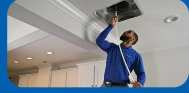
Duct Cleaning Services
